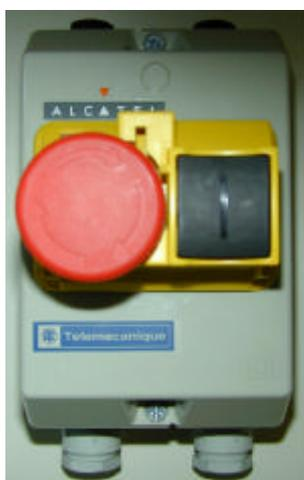
This device is intended to switch off the pump power. It also has one relay contact (1 normally open) for external use.
